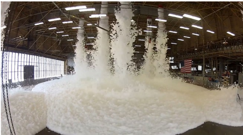
Abb. 6: Hangar der US Air Force, der für Testzwecke mit AFFF geflutet wird. 17 Originaltext: PFAS appears in firefighting foam that has been routinely used on military bases nationwide Foto: Department of Defense
